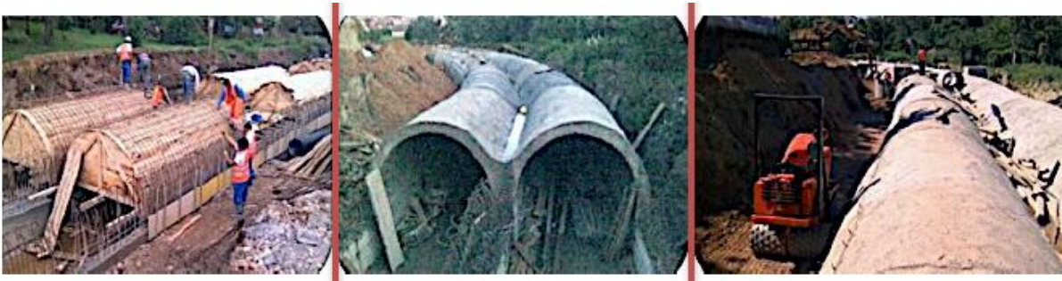
Fig. 7. Building, covering of river Prishtevka. (Source: Public Domain, 2012)
