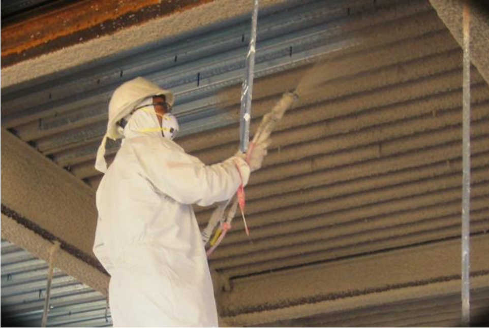
Fig. 3. Spray applied fireproofing
