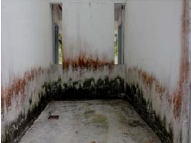
Figure 8: Fungi on external wall
