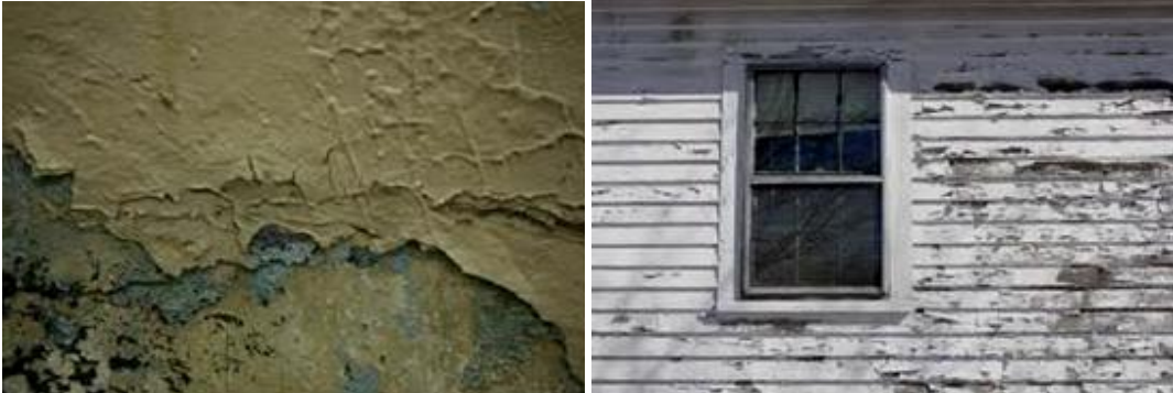
Figure 4: Peeling Paint
